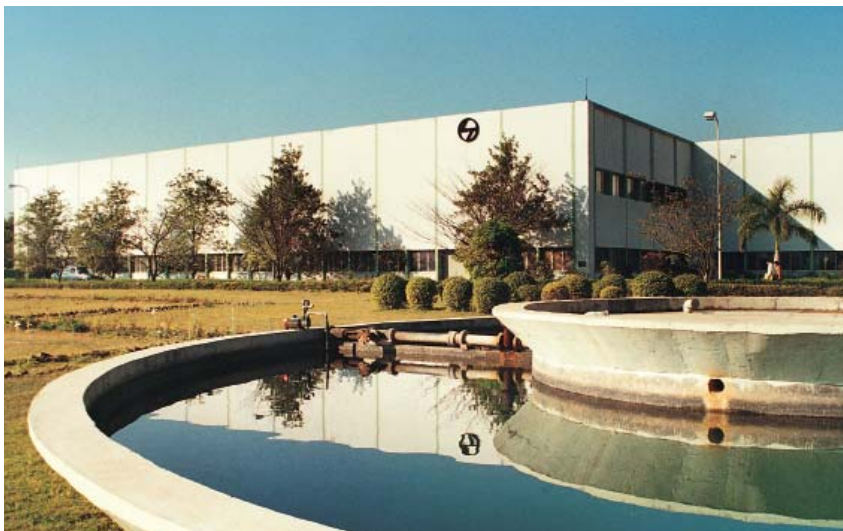
Switchgear Factory, Ahmednagar
