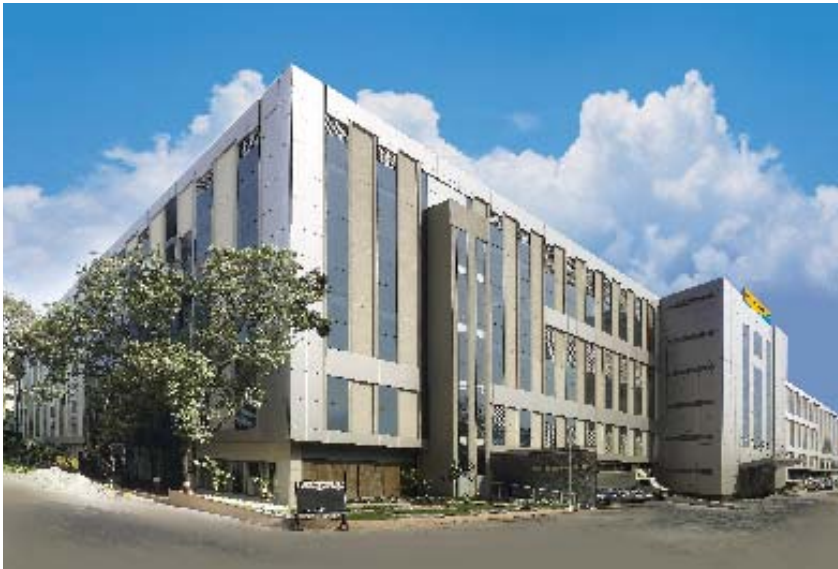
Switchgear Factory, Mumbai
