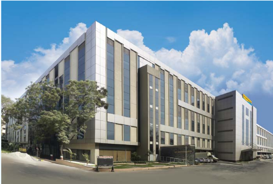
Switchgear Factory, Mumbai
